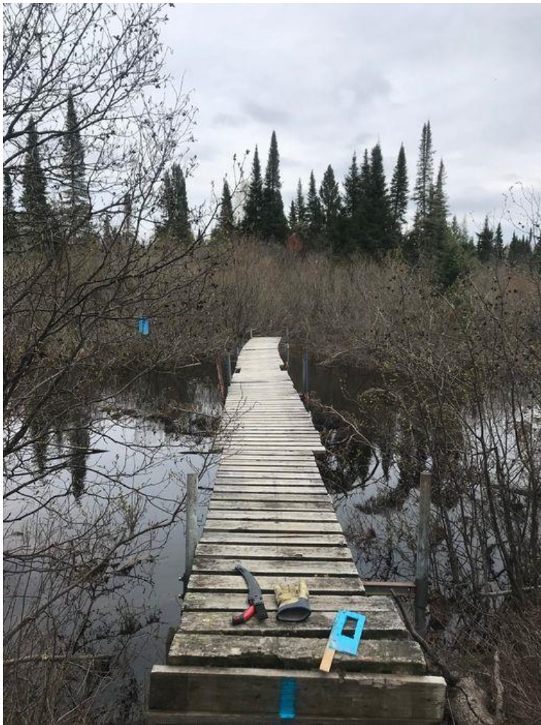
Stump River Bridge
